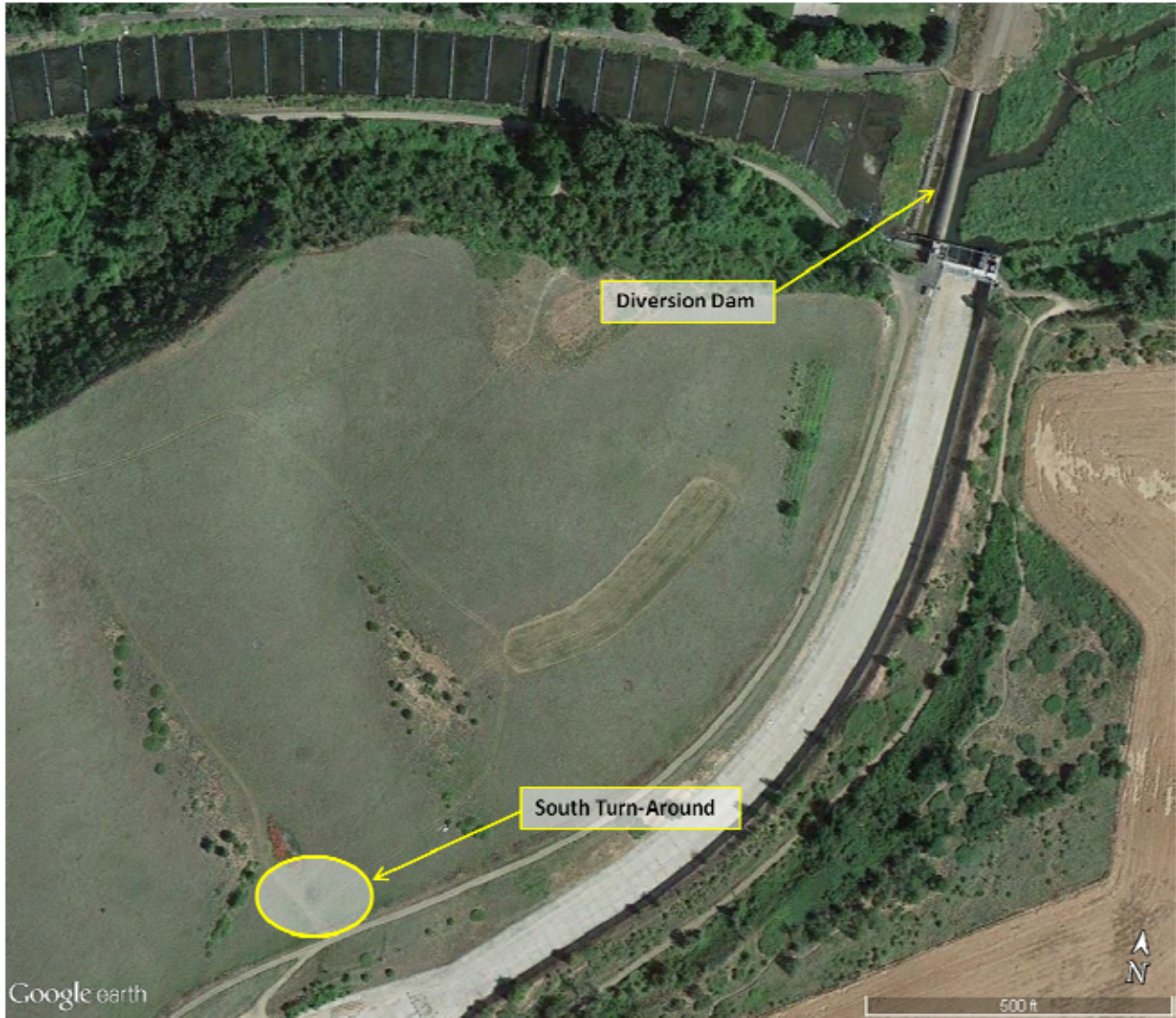
Figure 2-4: South Levee Turn-Around Site
