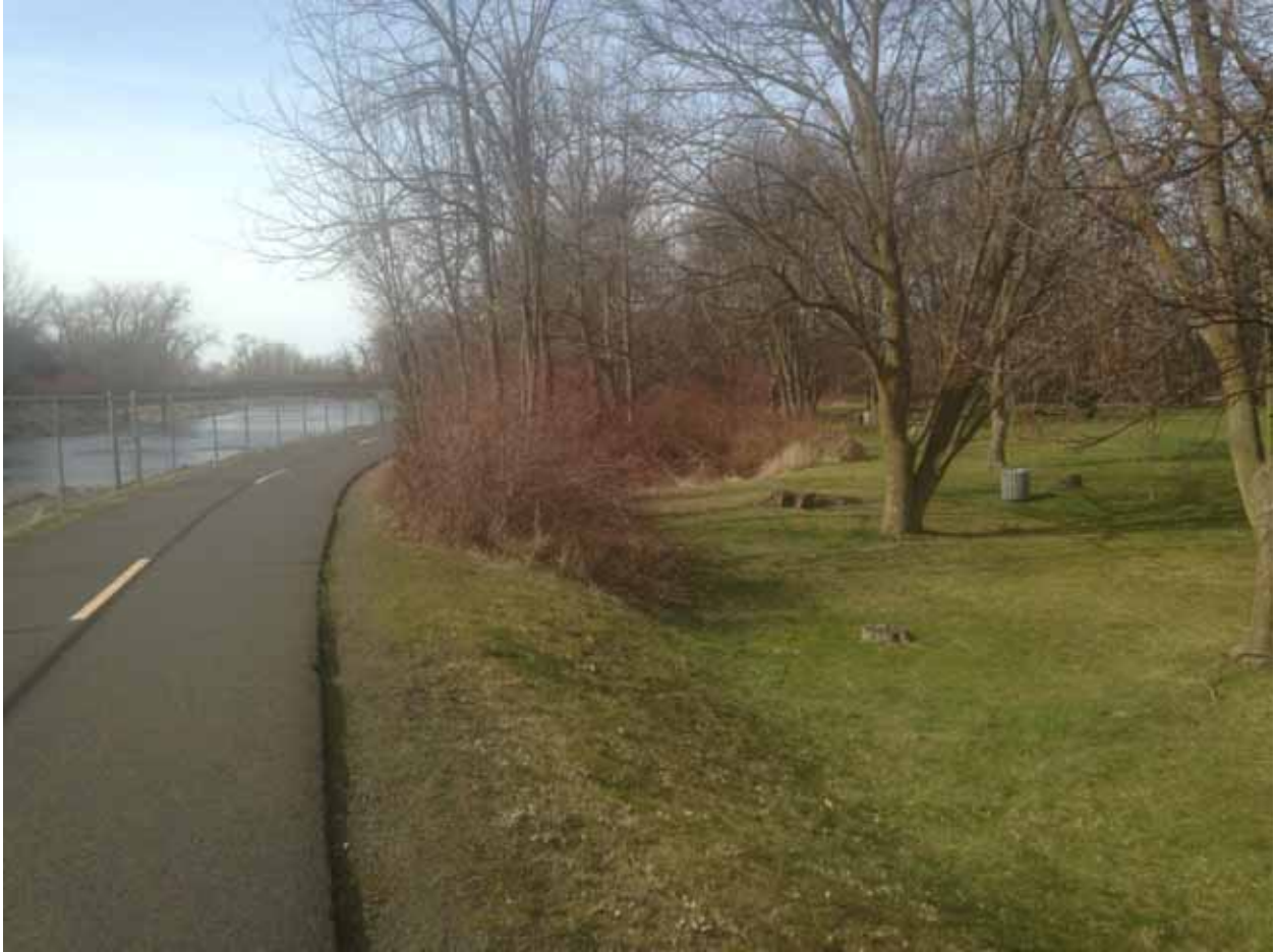
Photo 3-1: Vegetation Growing on the North Levee Structure at Rooks Park (Viewing West)
