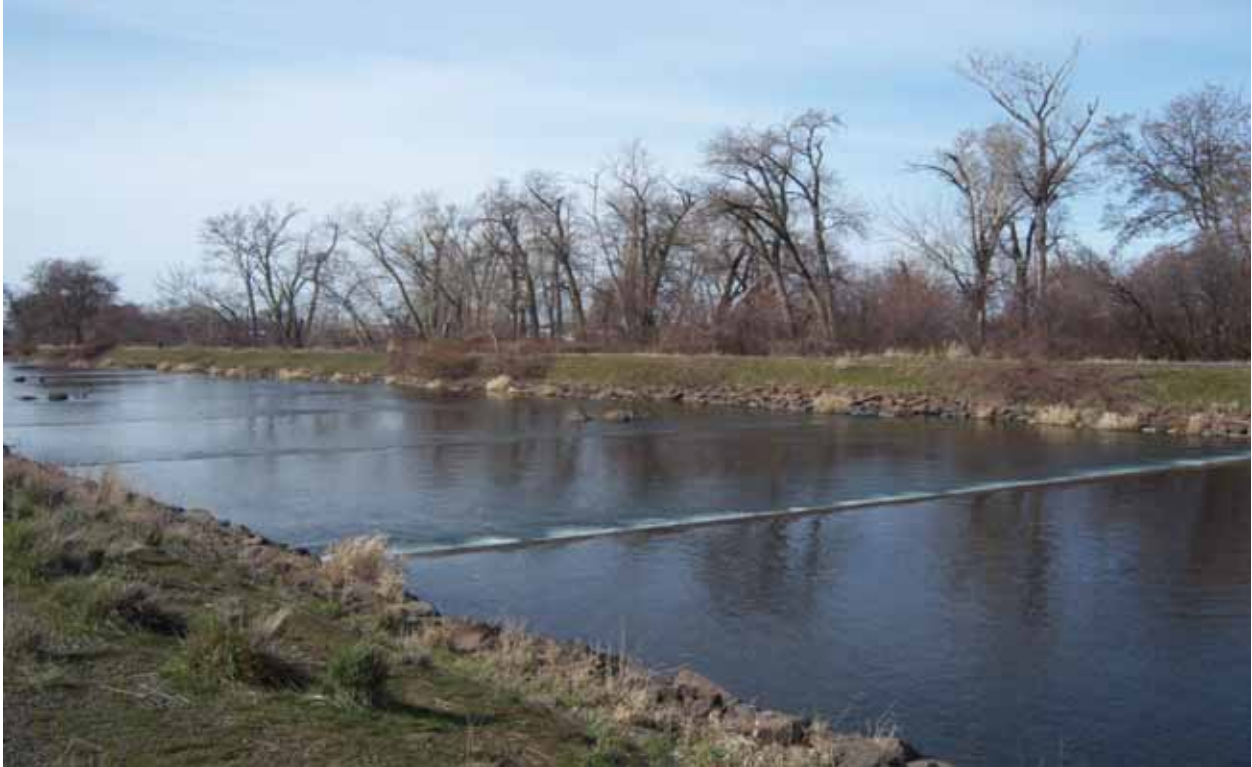
Photo 1-1: A Portion of the Federally-Owned Mill Creek Flood Control Project, Lined with Levees and In-Water Concrete Sills (Viewing West Northwest)
