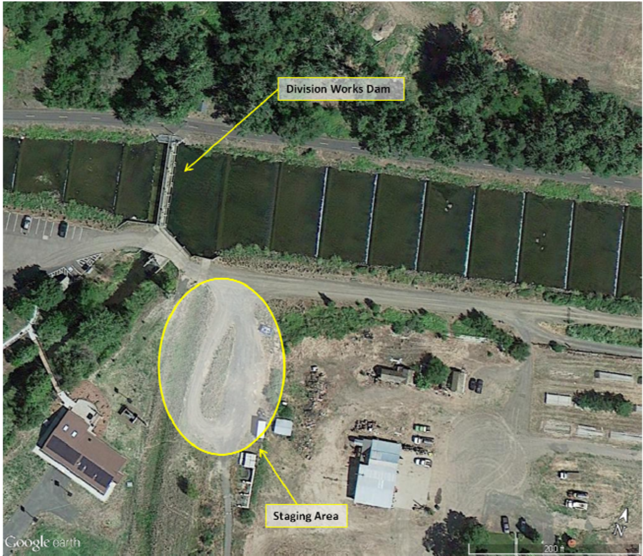
Figure 2-5: Horse Trailer Parking Area To be Used as a Contractor Staging Area
